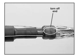
Stretch and tear off the end of the rubber mastic as shown.
