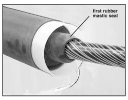
2.7.2 Continue to install the cold shrink tube over the rubber mastic on the other cable by slowly pulling and unwinding the outer core counterclockwise. This portion of the cold shrink tube installs differently than typical cold shrink products in that as the tube shrinks, the end rolls under. The tube may need a slight push to get over the second mastic seal.
