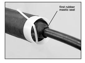
2.5.3 Continue to install the cold shrink tube over the rubber mastic on the other cable by slowly pulling and unwinding the outer core counterclockwise. This portion of the cold shrink tube installs differently than typical cold shrink products in that as the tube shrinks, the end rolls under. The tube may need a slight push to get over the second mastic seal.
