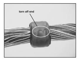
3.1.2 Begin to install the cold shrink tube by completely covering the rubber mastic, and slowly pulling and unwinding the inner core counterclockwise toward the splice body. The outer core should remain relatively stationary while unwinding the inner core. If the outer core begins to move towards the first mastic seal, gently pull the outer core and jacketing tube towards the second mastic seal and continue unwinding the inner core.
