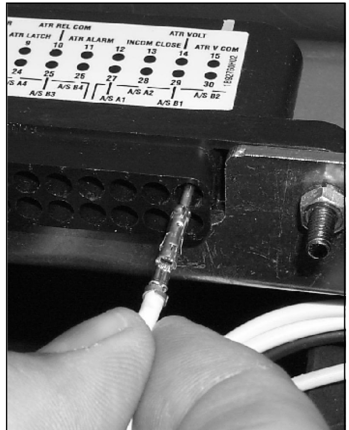
Figure 7. Wiring Secondary Block "A".
