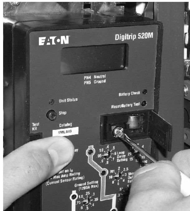
Figure 4. Loosening the Rating Plug Retaining Screw.
