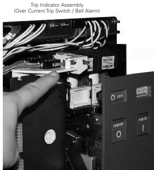
Figure 6. The Trip Indicator Assembly.
