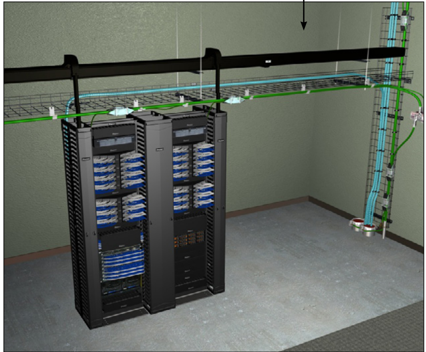
GACB-2 installed on Wire Basket System
